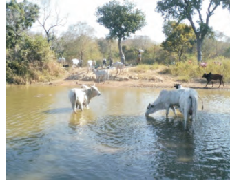
Agropastoral dam at Fombawi in the northern Benin
